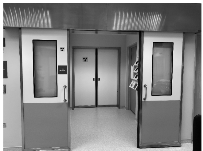
Fig. 2. Entrance to the patient anteroom. The outer set of inter-locking doors are currently ajar and this prevents the inner set of doors from opening.
