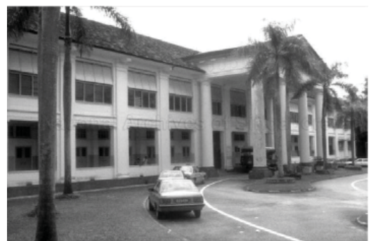
Fig. 2. Norris Block (Lower Block), Sepoy Lines General Hospital.
